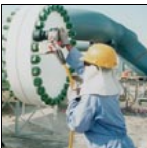
◀ Easy and reliable service in the field using Enerpac hydraulic wrench pumps and torque wrenches.
