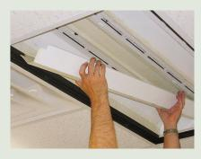
Leave the fixture housing and wiring in place to reuse with the new kit. Keep the space clean by not removing the ceiling tiles.
