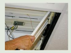
Upgrade internal fixture components with relight assembly containing fewer, longer-life lamps – and reduce your energy use by as much as 67%.
